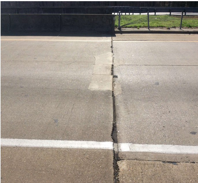
PHOTO 1 Description Bent 1 Joint bad
