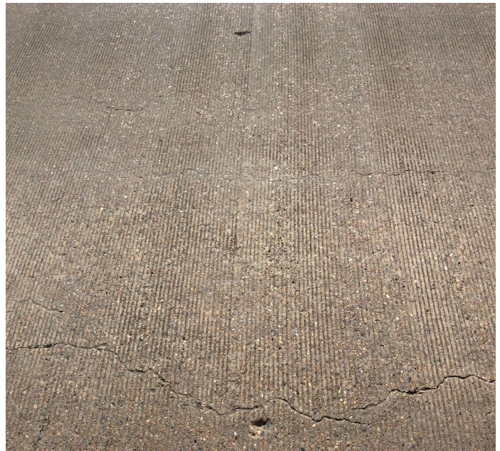
PHOTO 2 Description Sealable deck cracks...
